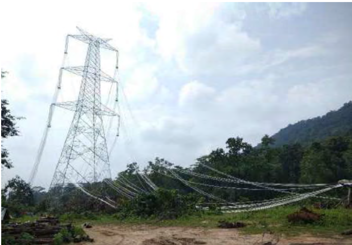
Stretch 115/6 to 116A/0 – Stringing in progress
