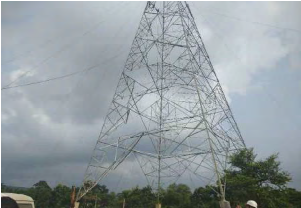
Location 108/3 – Tower erection in progress
