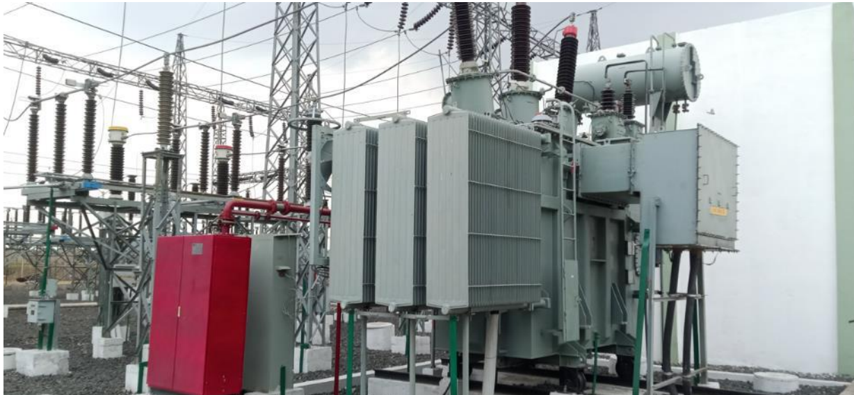
Figure 32: Power transformer
