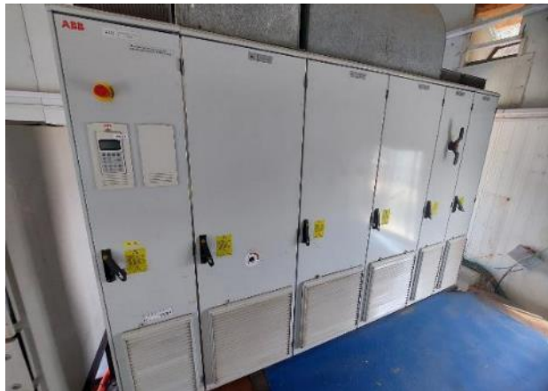
Figure 6: Inverter
