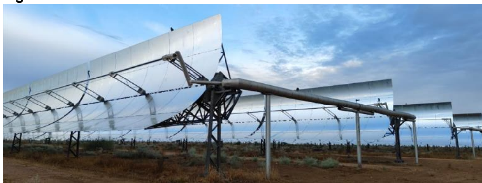
Figure 82: Solar PV collector
