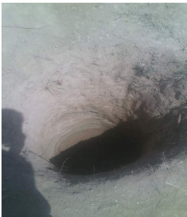
Visual identification of soil at 400/220 KV GIS Sub-station at Khor Pattan, Baramulla
