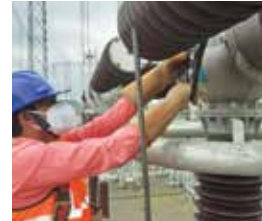
Switchyard Maintenance at Dhule Substation
